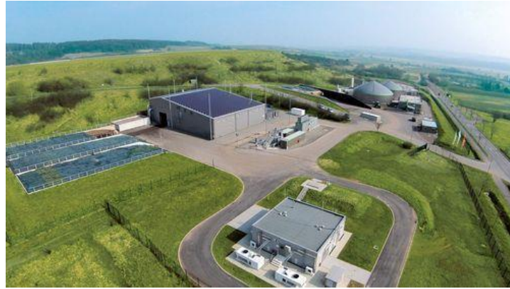
Figure 19: Pilot plant at Allendorf (taken from [14])
